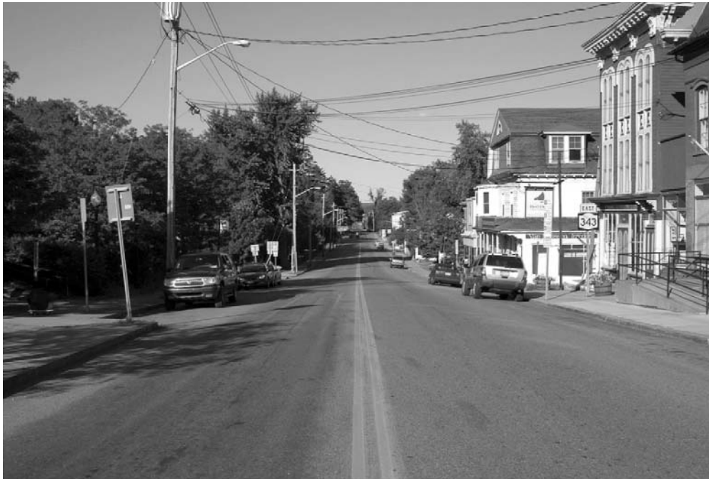
Existing View East on Main Street
