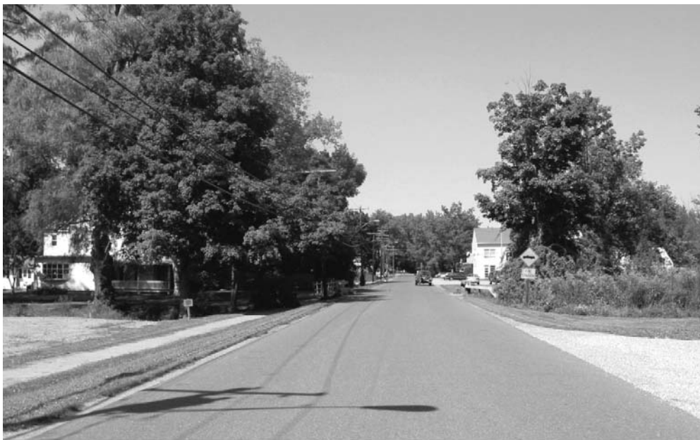
Existing View North on Mechanic Street near Stream
